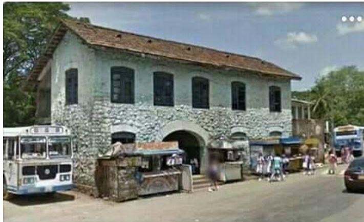
Figure 3.29 : Kahawatta Railway Station
