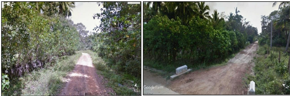
Figure 8_Conditions of internal Roads
