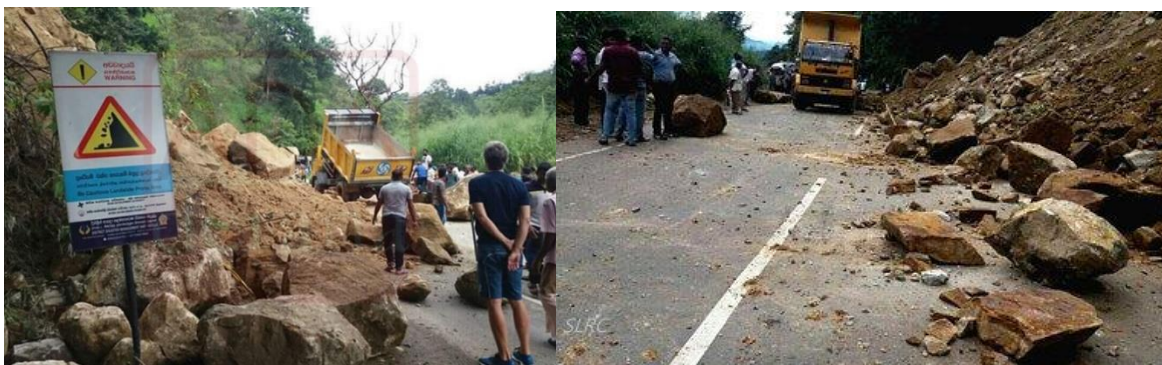
Figure 2.4 Ella Wellawaya Road – Landslides
