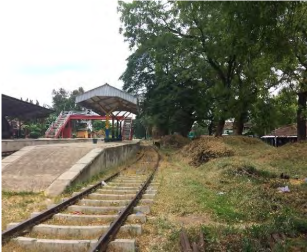
Existing condition of Wellawa railway station
